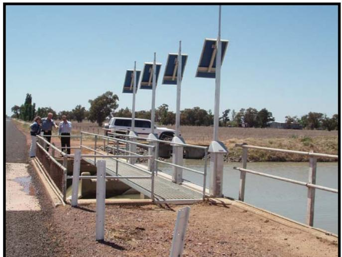
Remotely actuated gates of the Coleambally Irrigation Cooperative in New South Wales. This site is solar powered.
