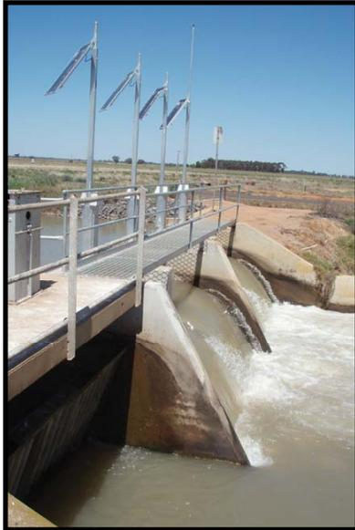
A sharp-crested weir flow condition allows these remotely actuated gates to be used for accurate flow measurements. The gates will automatically move to maintain a water surface level or to maintain a preset flow.
