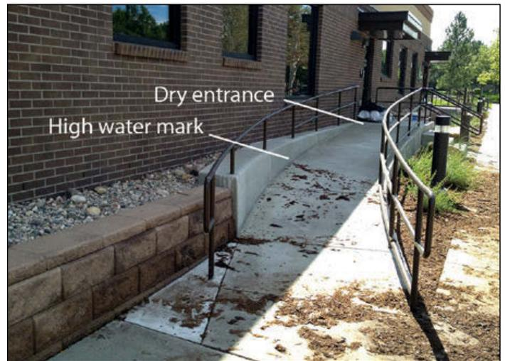
*Figure 2. Debris line is evident on west side of Orthopedic Center of the Rockies showing the water level against the building. Approximately 6 inches of freeboard remained before water would enter the building, making this a good example of the benefits of elevating structures to protect from flood damage.*
