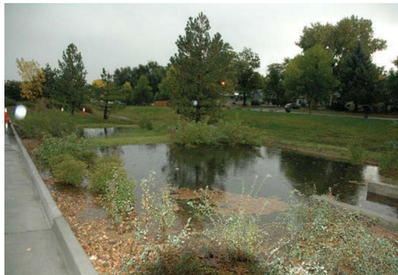
Figures 3 and 4. Bioretention cell installed in Fort Collins, CO during dry and wet weather. Bioretention cell treats stormwater runoff from an adjacent parking lot. Photos by Chris Thornton
