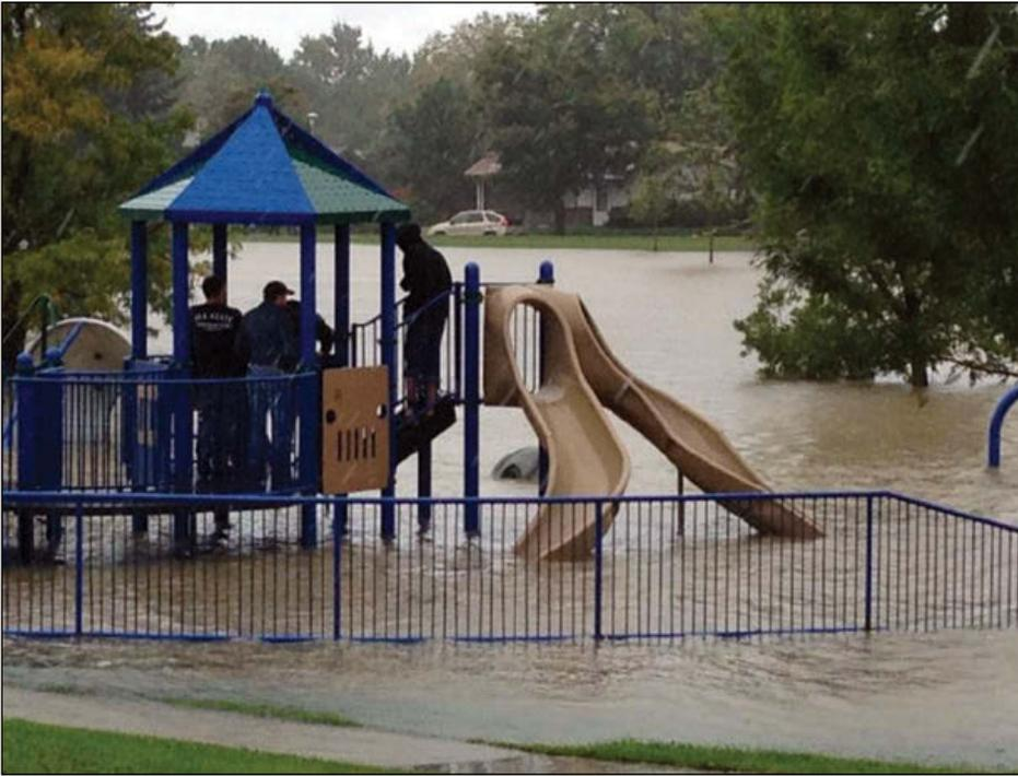
Utah Park in Aurora, Colorado is a detention basin that worked as designed to minimize damage from floodwater to neighboring property during the September, 2013 flooding. Photo by Jeremy Deischer
