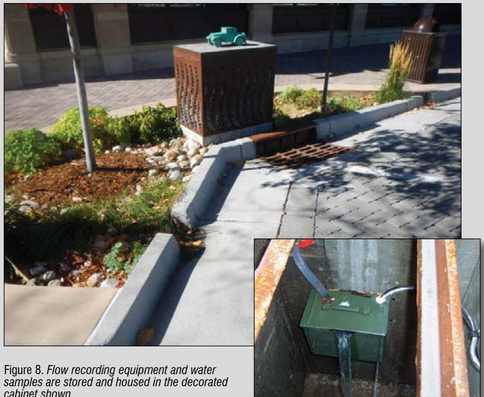
Figure 8. *Flow recording equipment and water samples are stored and housed in the decorated cabinet shown.*
