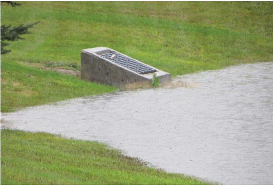
Figure 2. Properly maintained outlet with no noticeable pollutant or trash buildup. Photo by Larry Roesner
